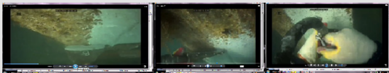
Figure 4: The method of applying epoxy-coating under water.
